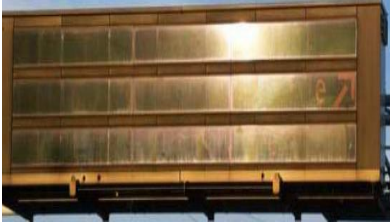
Figure 15. VMS Visibility Degradation due to Sunlight [10]
