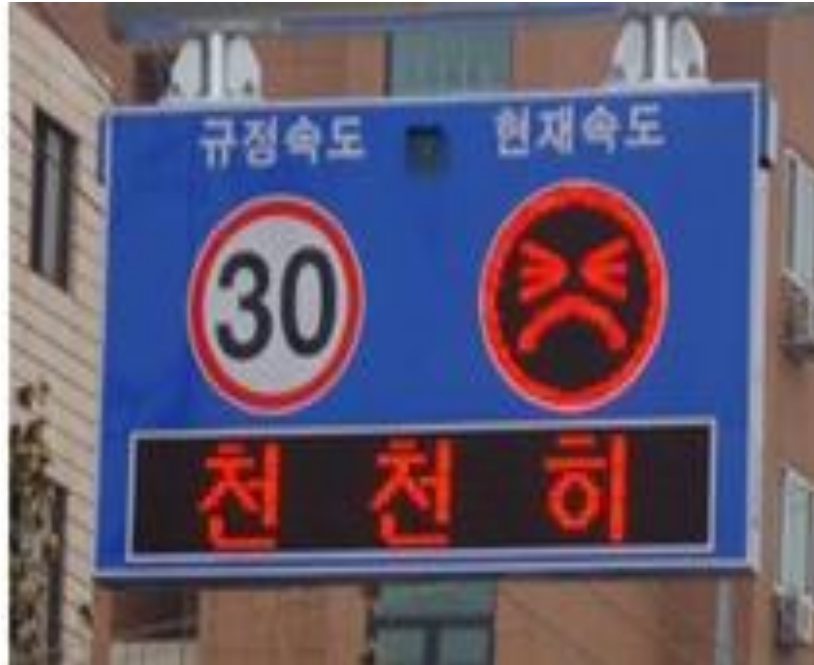
Figure 1. Variable Message Signs Installed in Children Protection Zones in Nowon-gu and Yangcheon-gu in Seoul [2]
